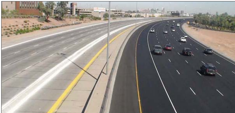
The attractive qualities of R-A verse cement asphalt (Arizona's I-10 Freeway)
